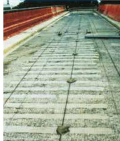
Carboplate covered with Mapegrout BM
