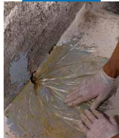
The splayed end of a piece of MapeWrap FIOCCO
