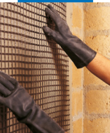
Positioning of Mapegrid G 220
