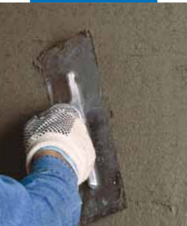
Covering Mapegrid G 220 with a further layer of Planitop HDM
