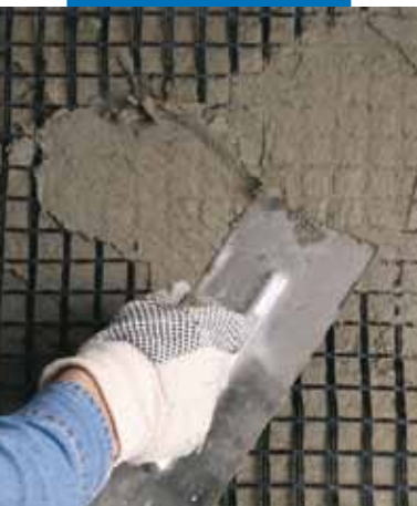
Positioning of Mapegrid G 220
