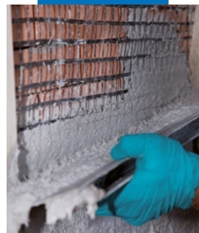
Application of Planitop HDM Restauro system with Mapegrid G 220 on a brick wall
