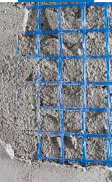
Structural render made using Planitop SR and Mapenet EM 40
