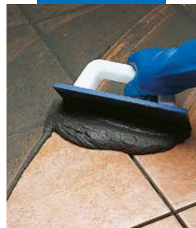
Grouting single-fired tiles with a float
