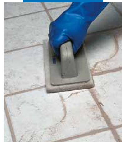
Finishing with a Scotch-Brite® pad
