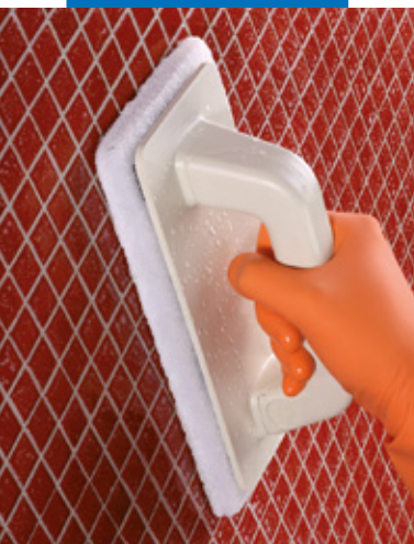
Cleaning off the glass mosaic with a damp Scotch Brite® pad
