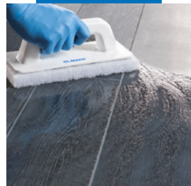
Cleaning the joints with a Scotch-Brite pad
