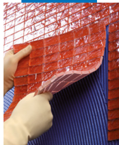
Laying glass mosaic with Kerapoxy Design on wall
