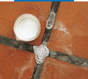
Cleaning an efflorescence
