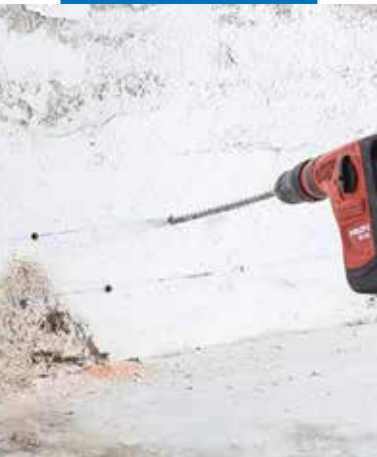
Drilling the holes
