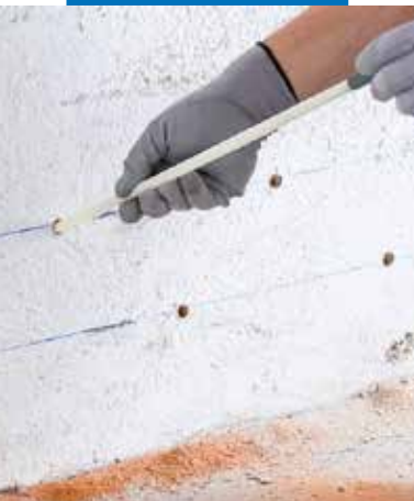
Inserting the injectors in the holes
