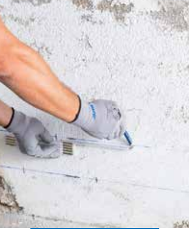
Preparing the holes
