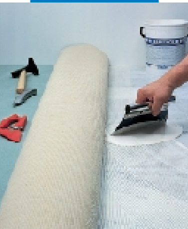
Laying carpet with Mapetack
