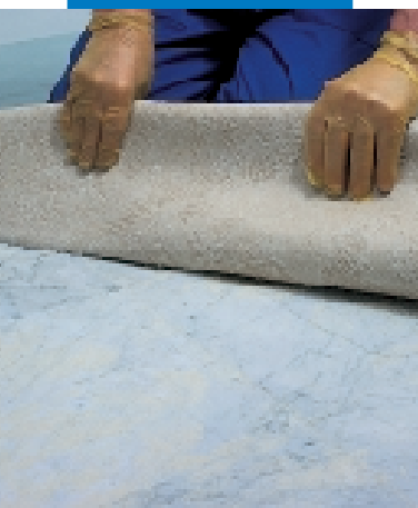
Removing carpet installed with Mapetack
