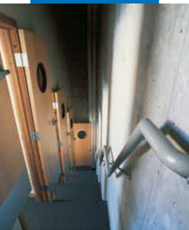
Example of carpet laid on a stairway - Judges Tower for the ski-jumping event at the 2002 Salt Lake City Winter Olympic Games - USA
