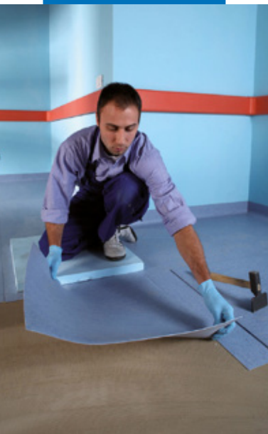
Installing PVC floor tiles
