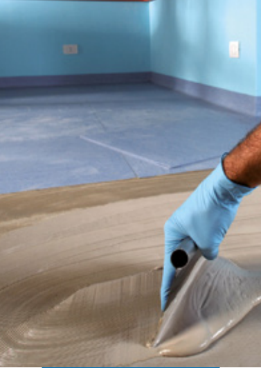
Applying Ultrabond Eco 380
