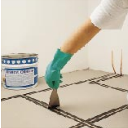
Setting the copper wire with ADESILEX VZ CONDUCTIVE
