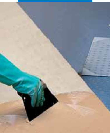
Installing rubber flooring with Adesilex G12
