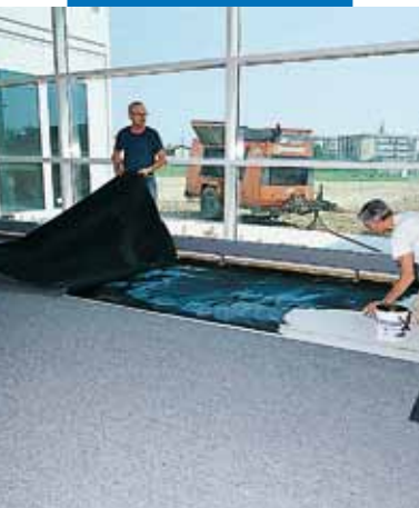
Installing industrial flooring in an electronics company
