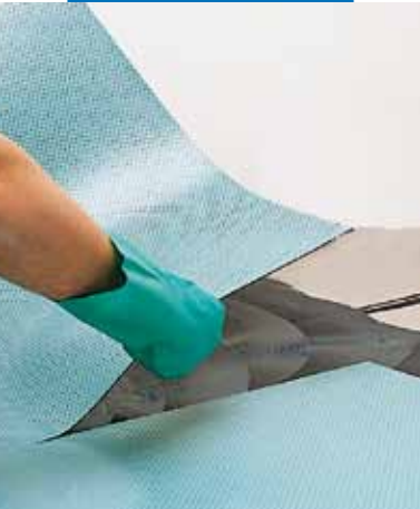
Laying conductive PVC tiles
