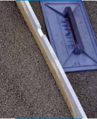
Evening off the substrate made with Mapedrain Mortar
