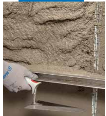
Levelling MapeWall Inject & Consolidate with a straight-edge
