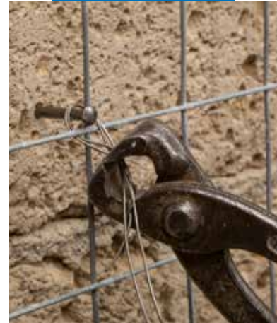
Fastening the metallic mesh in place
