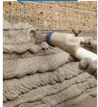
Application of MapeWall Render & Strengthen with a rendering machine
