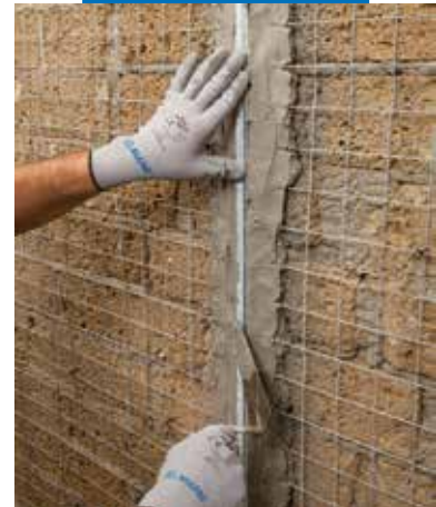
Placing the vertical guides in place
