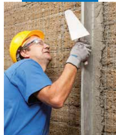
Checking that the vertical guides are plumb
