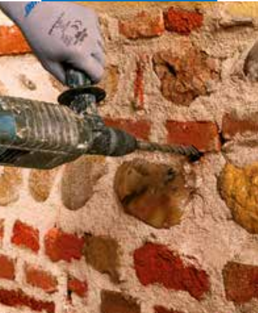
Preparing the holes for Mapenet EM Connector
