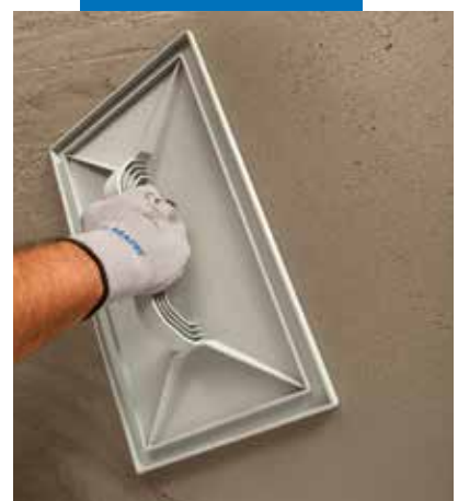
Levelling the substrate
