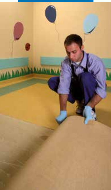
Installing linoleum sheets with natural jute back
