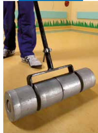
Rolling linoleum flooring
