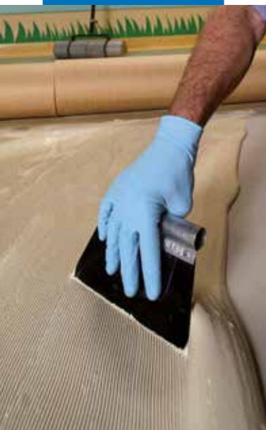
Applying Ultrabond Eco 520
