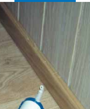
A wooden skirting applied with Ultrabond Eco 575
