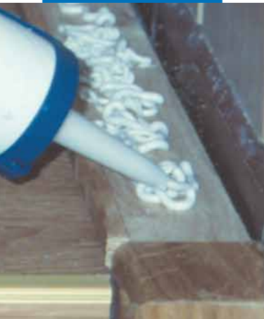
Bonding a wooden skirting with Ultrabond Eco 575
