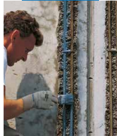
Application of Mapefer
