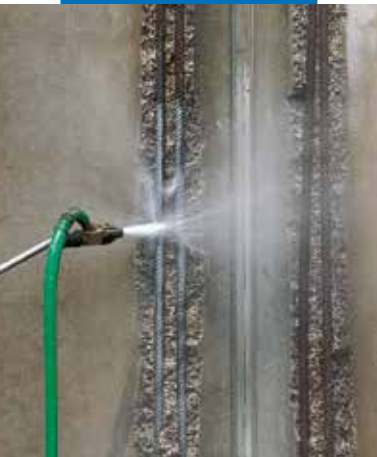
Cleaning reinforcing rods with hydro-sandblasting
