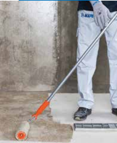
Application of Primer SN on the substrate
