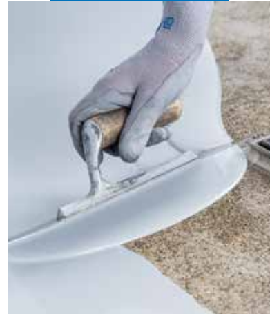
Application of Mapegum EPX
