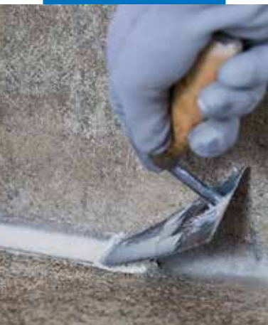
Forming fillet joints
