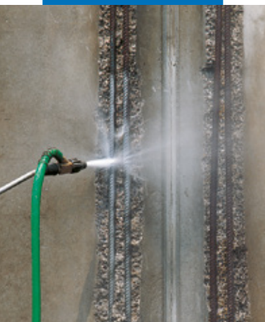
Cleaning reinforcing rods
