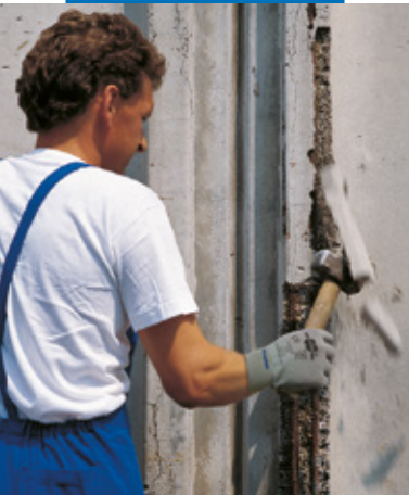
Demolition of degraded concrete
