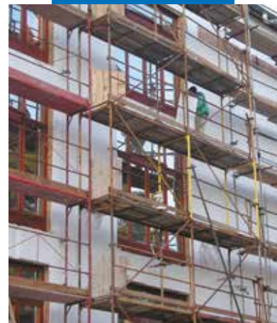
Bonding the insulating blocks to the façade with Mapetherm AR1
