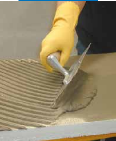
Applying Mapetherm AR1 on the back of the panel with a notched trowel
