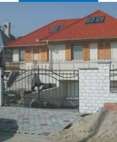
Private villa with foamed heating insulation - Hungary
