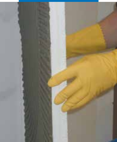
Installing the insulating panels
