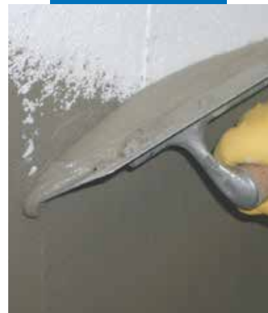
Smoothing insulating panels: spreading the Mapetherm AR1
