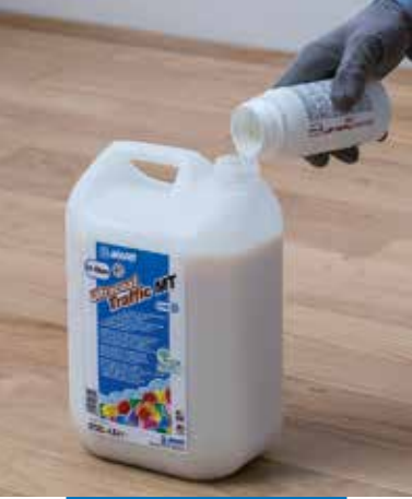
Mixing component A directly in the drum
