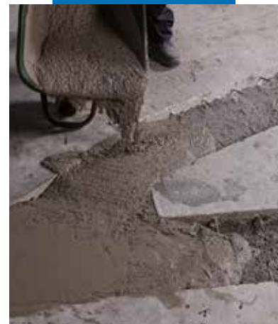
Application of Mapegrout SV Fiber in the area under repair
