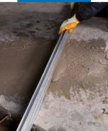
Levelling off Mapegrout SV Fiber with a straight-edge
