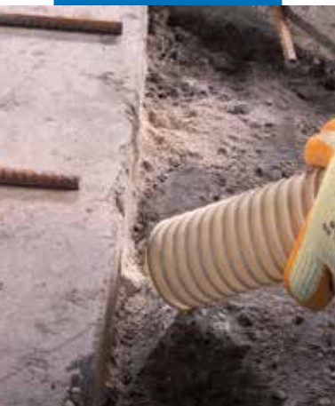
Removing dust with a vacuum cleaner
