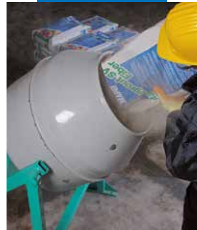
Preparation of the Mapegrout SV Fiber mix
