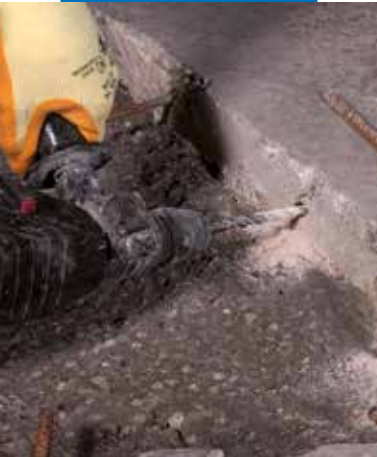
Preparation of the holes to insert the reinforcement rods (dowelling)
