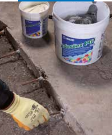
Fixing reinforcement rods for the dowelling in place using Adesilex PG1
