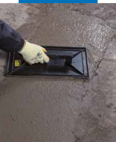
Tamping Mapegrout SV Fiber
