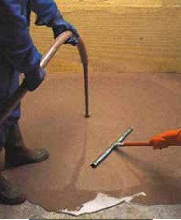
Application of Ultraplan with pump and squeegee
