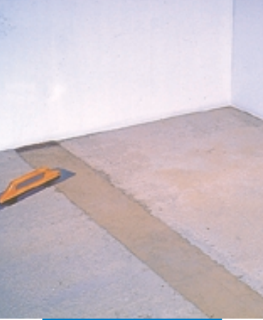
Substrate that needs levelling
