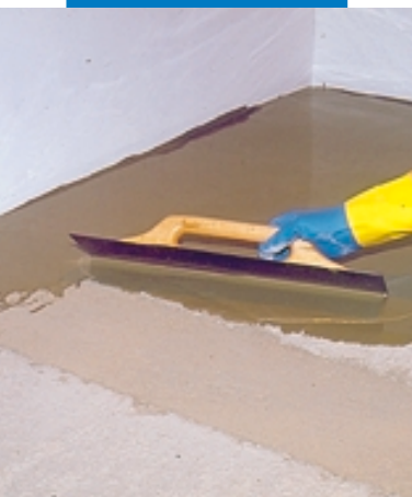
Applying Planolit with a trowel
