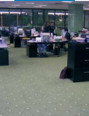
Installation of textile flooring on a substrate levelled off with Pianocem M mixed with water and Livigum. Olio Carli SpA - Oneglia (Imola) - Italy
