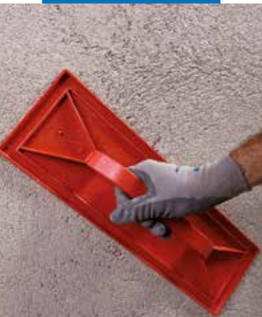
Levelling the surface of Mape-Antique MC
