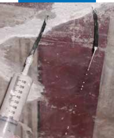
Injecting Mape-Antique F21 into a frescoed wall
