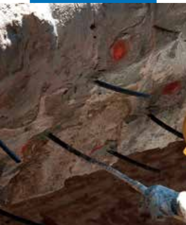
Injecting Mape-Antique F21 into a stone masonry
