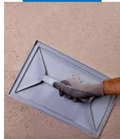
Levelling the render
