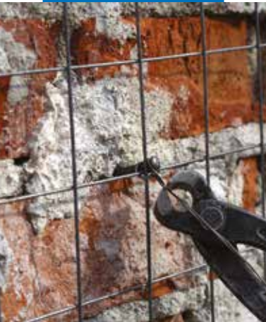
Fastening zinc-plated mesh to the masonry
