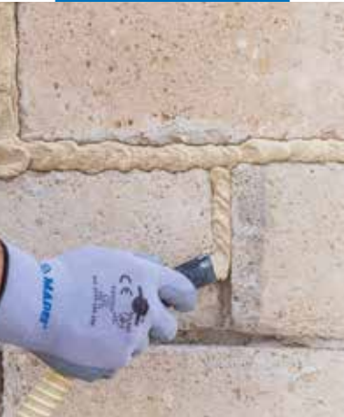
Removing the excess mortar
