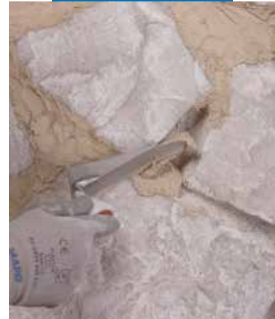
Pointing the joint in a stone wall
