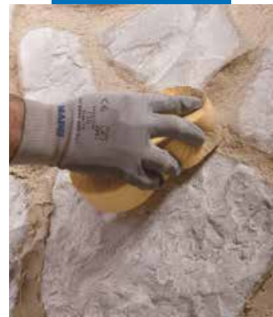
Finishing the surface with a sponge
