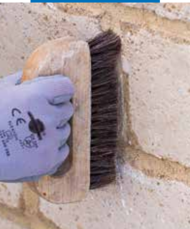
Finishing the mortar joints
