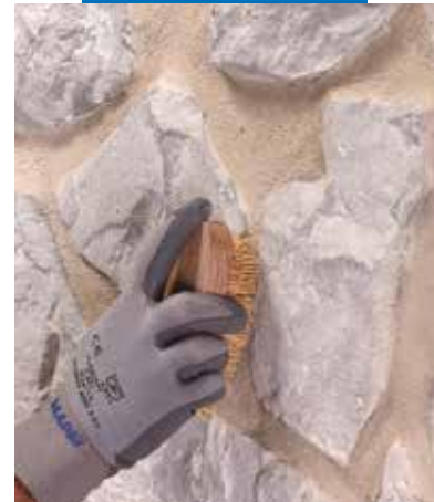
Finishing the surface with a millet brush
