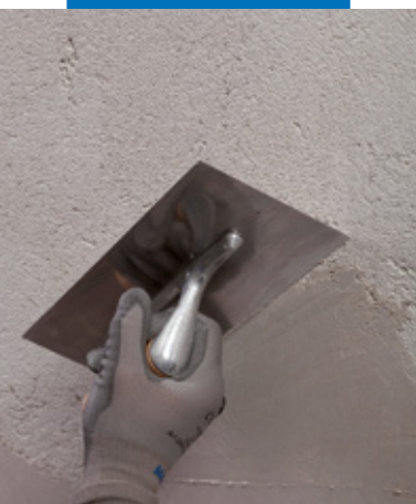
Application of Mape-Antique FC Civile
