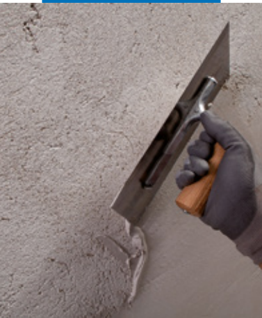
Application of Mape-Antique FC Civile
