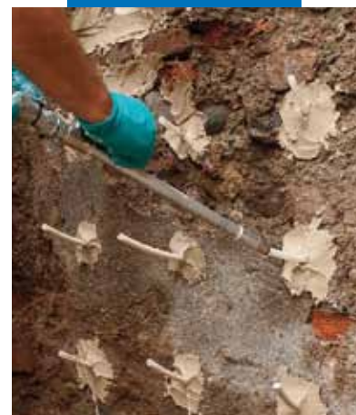
Injection of Mape-Antique I-15
