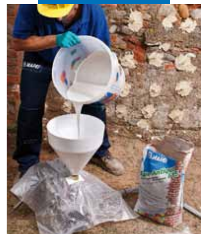
Filling the hopper with Mape-Antique I-15
