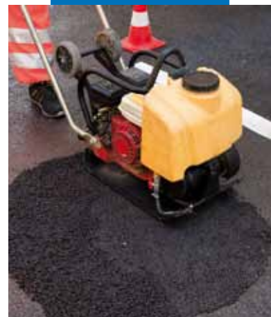
Compacting Mape-Asphalt Repair 0/8 with a vibro-compactor
