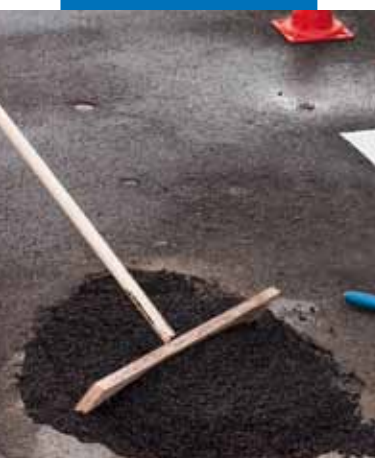
Applying and spreading Mape-Asphalt Repair 0/8
