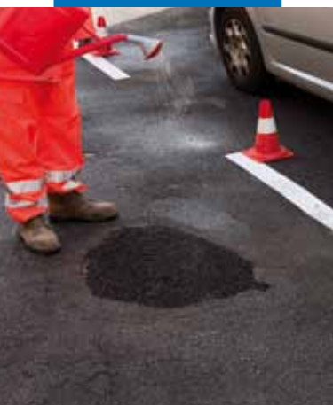
Wetting the surface of Mape-Asphalt Repair 0/8
