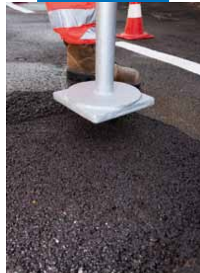
Compacting Mape-Asphalt Repair 0/8 by hand
