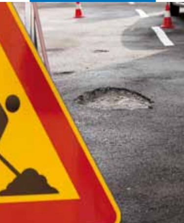
Road in a hole ready to be repaired
