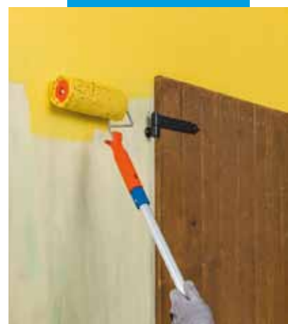
Application of Quarzolite HF Plus
