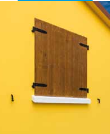
Façade repaired with Quarzolite HF Plus
