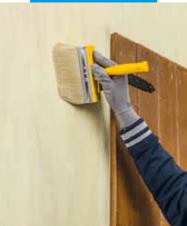
Application of Silancolor Cleaner Plus
