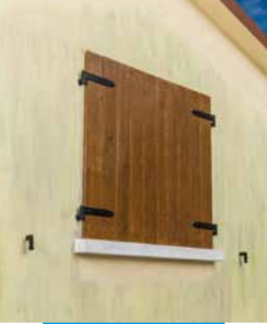
Façade damage by mould
