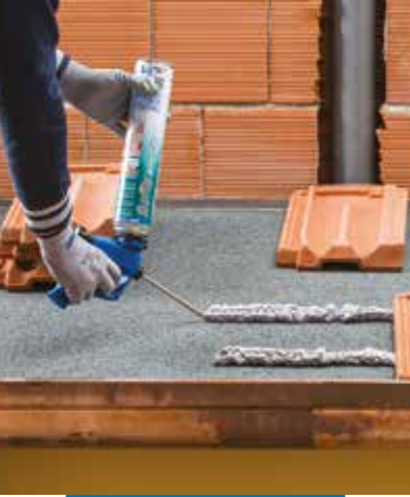
Bead-bonding roof tiles
