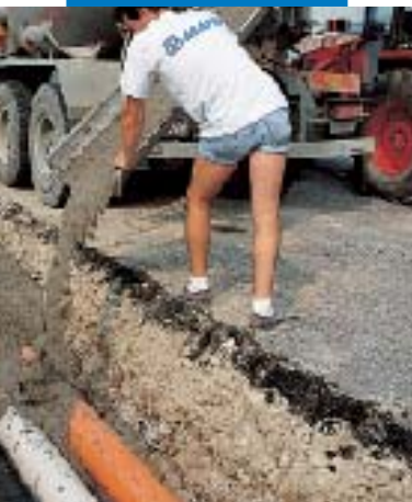
Unloading the foamed concrete from the mixer
