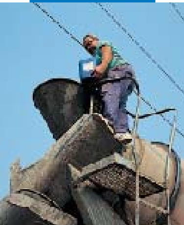
Pouring Mapeplast LA in to the mixer
