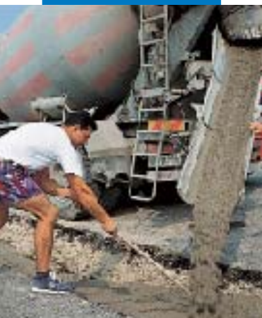
Levelling the foamed concrete
