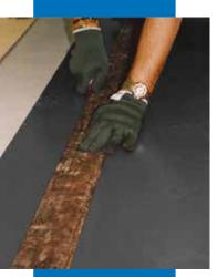
Cutting the joint between sheets of Mapelay
