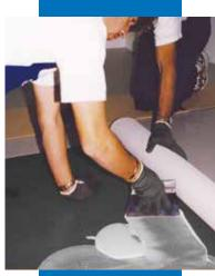
Laying rubber floor covering on Mapelay sheets using Adesilex G19. N.B. The joints between the sheets of rubber floorings are staggered with respect to the joints in the sheets of Mapelay
