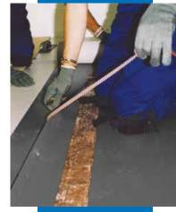
Removal of the cutted portion of Mapelay
