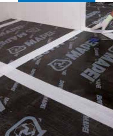
Once alignment of the Mapesilent Panel tiles has been checked, carefully seal all the joints using Mapesilent Tape
