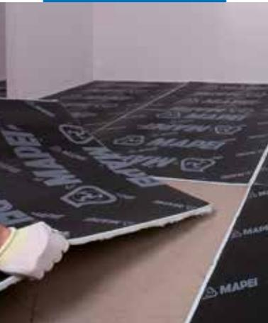
Lay the Mapesilent Panel tiles with the fibre layer (the light-coloured side) towards the bottom, making sure they are perfectly aligned
