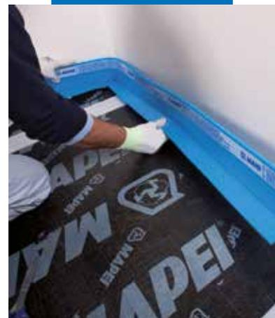
**Position the angle of Mapesilent Band R in order to check that the two sides of the cut match perfectly**
