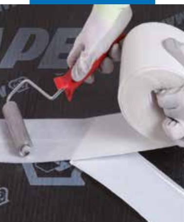
To guarantee that Mapesilent Tape bonds perfectly, we recommend passing over the surface of the tape with a rigid or semi-rigid roller
