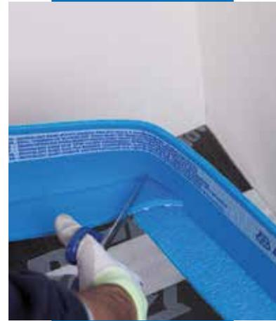
**Cut the lower part of Mapesilent Band R to form a 90° angle and remove the protective backing film to expose the adhesive part**
