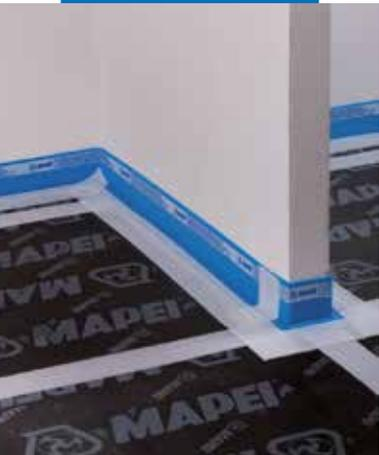
Once work has been completed, Mapesilent Tape must be visible on all the overlaps and joints of Mapesilent Panel and Mapesilent Band R. There must be absolutely no contact points with the substrate, to avoid the formation of acoustic bridges
