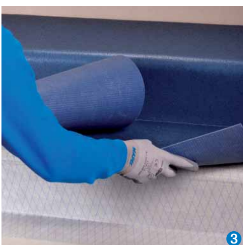
Application of PVC on steps using Mapecontact
