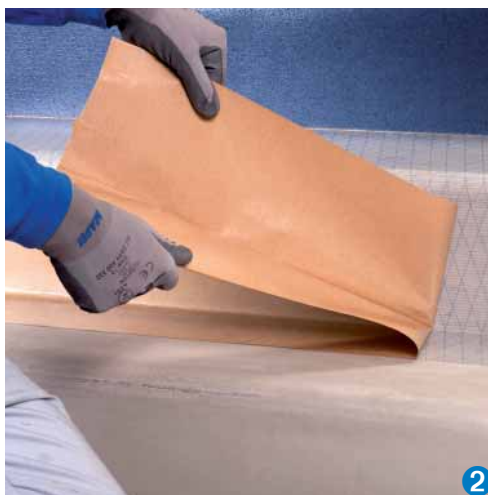
Removal of the protective coating
