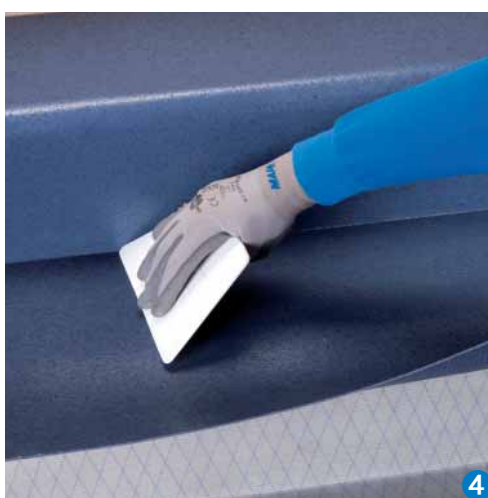
Massaging the PVC after applying Mapecoat
