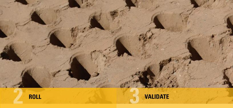
Compact the soil with vibratory system active, using the MDP value as your target.
