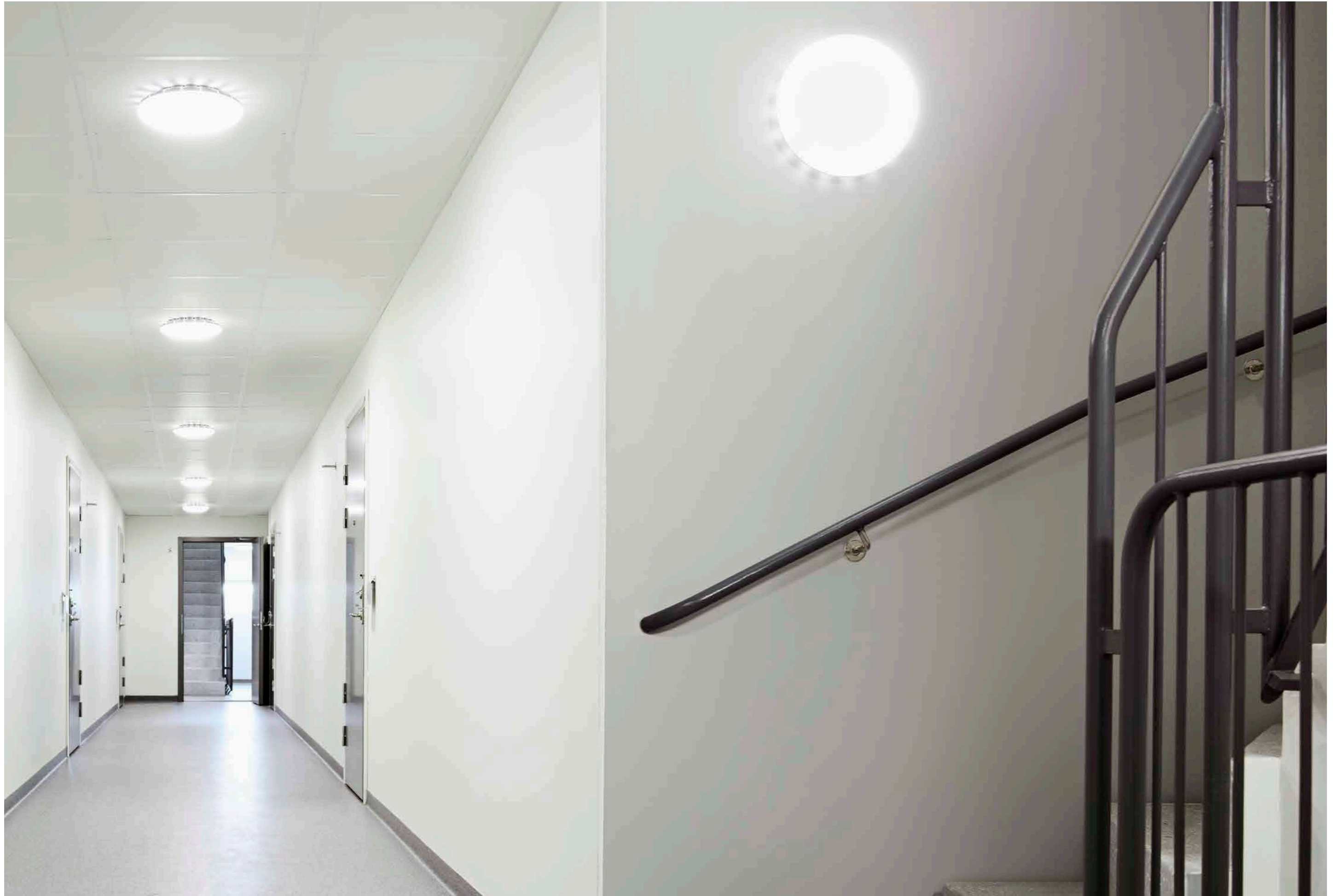
High-frequency sensor-switched light RS PRO LED S1 in the stairwells and corridors of the IKANO residential complex at Helsingborg, Sweden.
